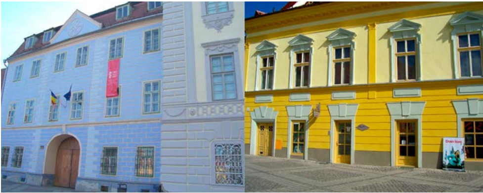
Figure 3. Renovated façades in Sibiu's historic center.
