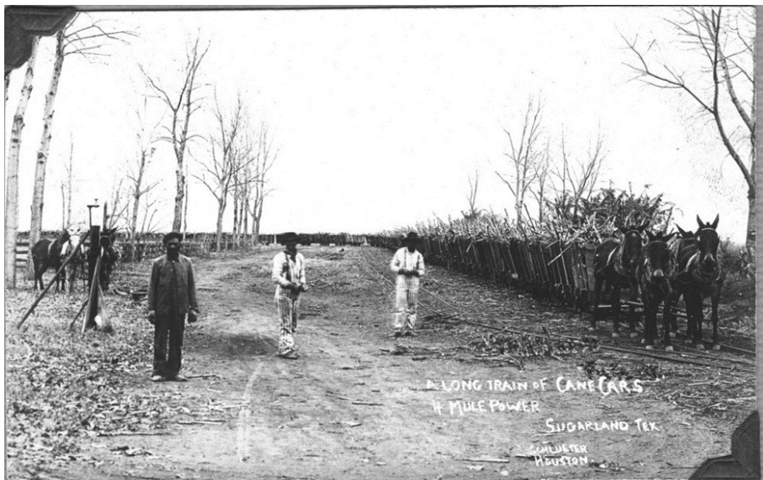
Figure 3: Convicts working near Imperial Farm, 1908. Crews would take portable rail car tracks and place them near cane harvesting areas. Cane would then be transported back to the nearest mill. Photo from Images of America: Sugar Land , Sugar Land Heritage Foundation. p. 14.
